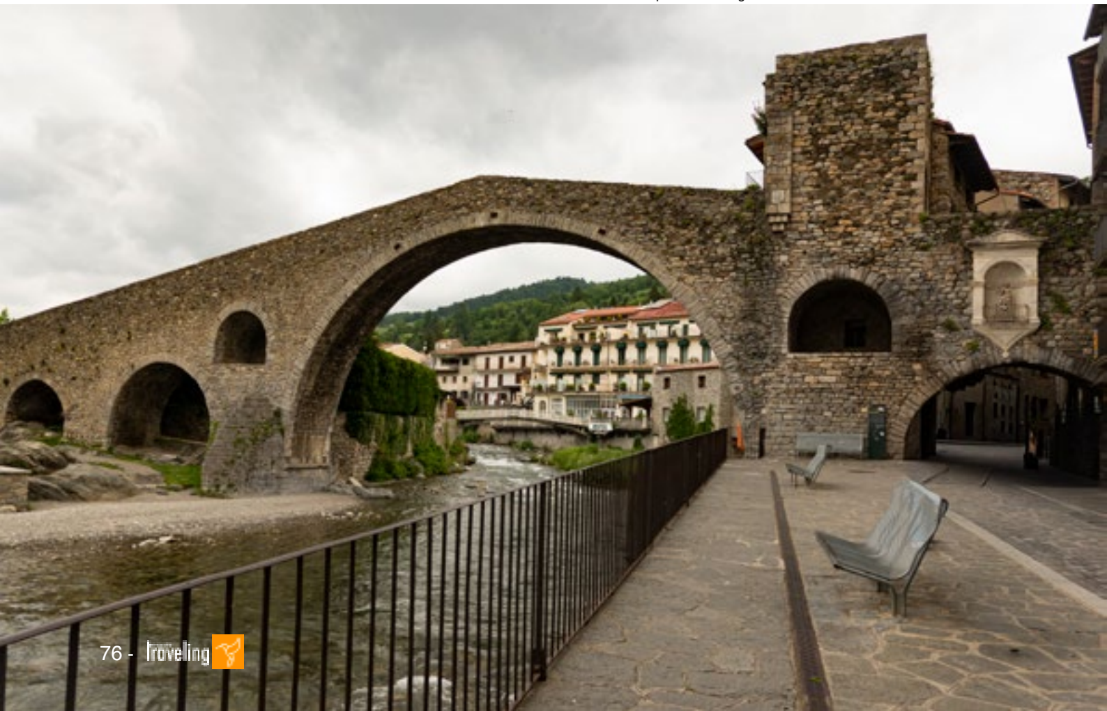
View of Campdorón's bridges
