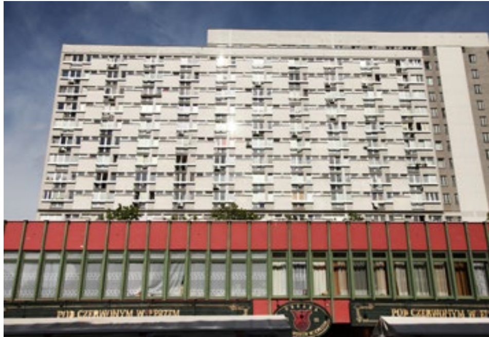
A socialist-era block of flats and the groundbreaking restaurant known as 'The Red Pig'
