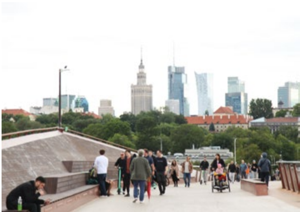
Magdalena Abakanowicz Footbridge over the Vistula River
