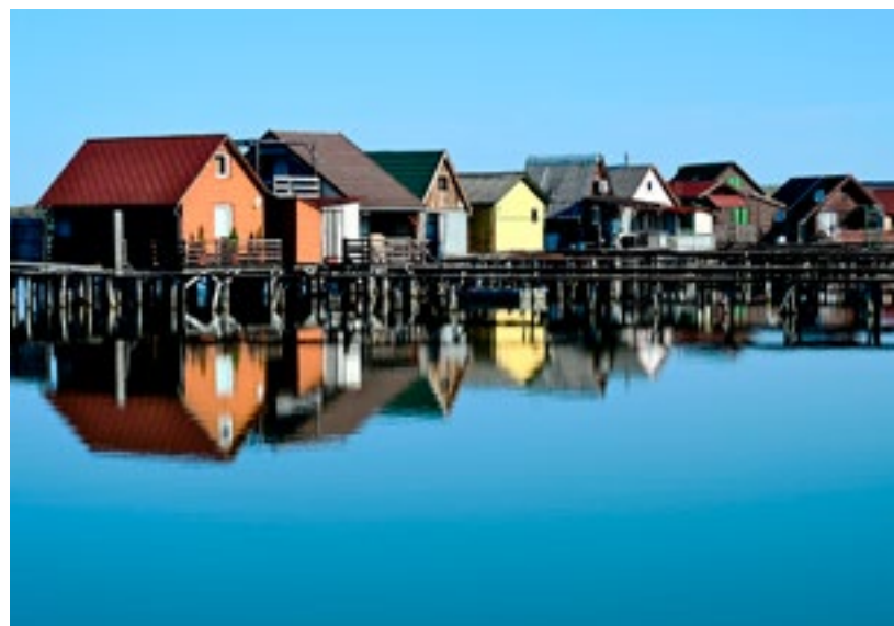
Panoramic view of the houses overlooking the lake
